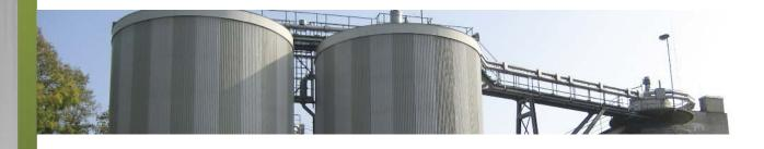
In order to gain a competitive advantage in the anaerobic digestion industry, Berlie Technologies Inc. has created a partnership with a German company to provide a high performance anaerobic digestion technology. Since 1994, this technology has been validated at large scale on municipal sludge and certain organic wastes. It allows for shorter treatment times (about seven days), compared with conventional anaerobic digestion processes (about twenty days).
