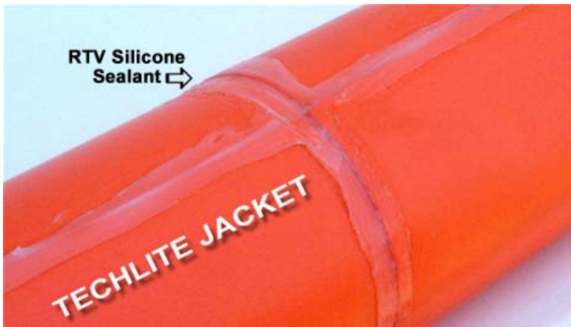
Photo 1: All seams over sealed with RTV
